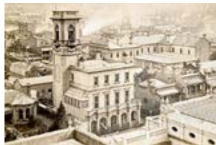
'Rostella' at 460 Lonsdale Street in the vicinity of the Supreme Court
